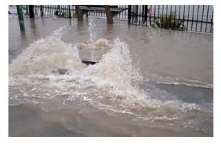
Photograph 3-6: Surcharging gully at Clifton Drive
