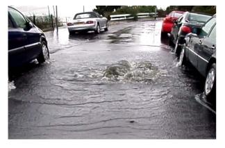
Photograph 3-5: Surcharging manhole at Clifton Drive
